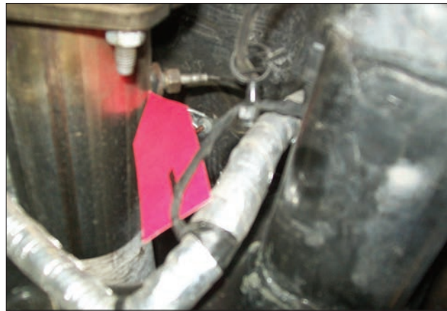
Arrow #1, EGT1 sensor in the exhaust pipe before the DOC/DPF housing
