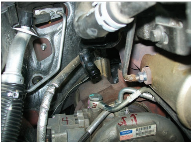
Arrow #1, turbocharger speed sensor under the foil cover for the wiring harness. Arrow #2, pressurized oil inlet to the turbocharger center housing. Arrow #3, coolant line. Arrow #4, VGT controller.
